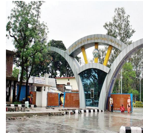
Strengthened RHFW (CHHEB, Kangra)
